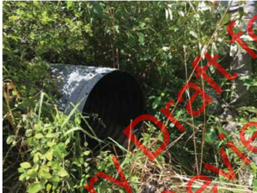
14 inch culvert South of railroad trestle.
