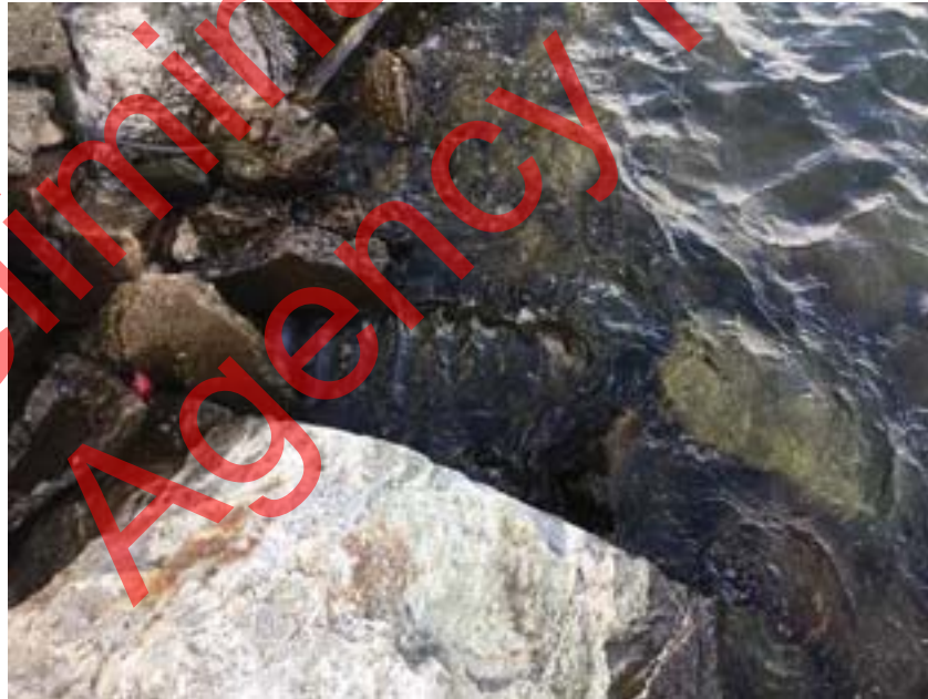
View of culvert.
