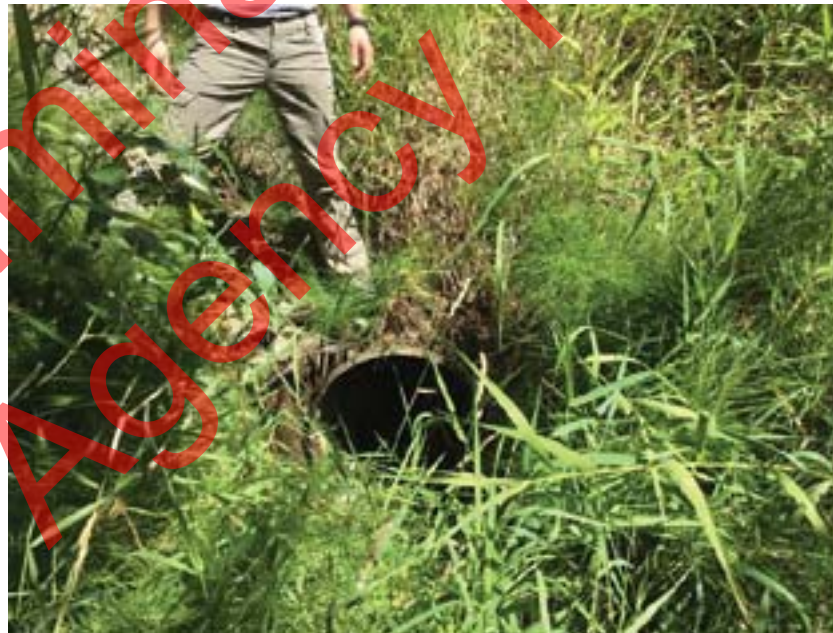
Facing east directly in front of culvert.
