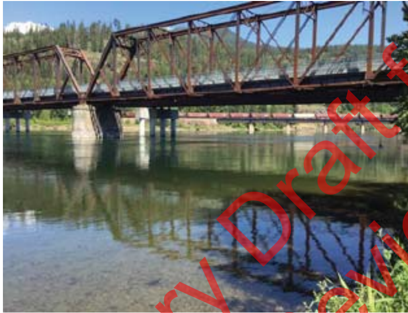
View looking upstream from collection point to River right bridge piling anchor.
