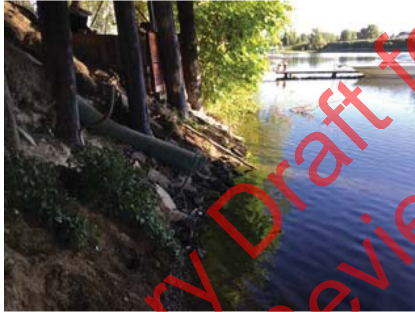
Image of concrete submerged culvert.
